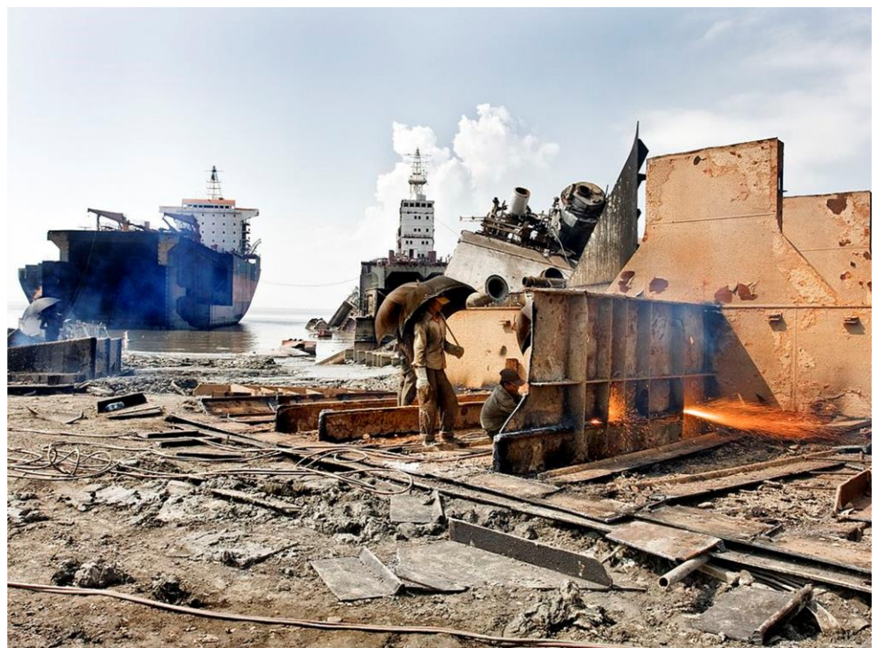
Ship Breaking by Gas Cutting in Bhatiary Yard 01, Chittagong Bangladesh. Photo by Naquib Hossain, CC BY-SA 2.0 https://creativecommons.org/licenses/by-sa/2.0 , via Flickr (N. Hossain, 2009)
